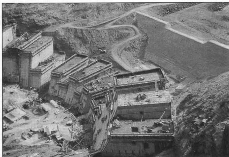
Katse Dam under construction
